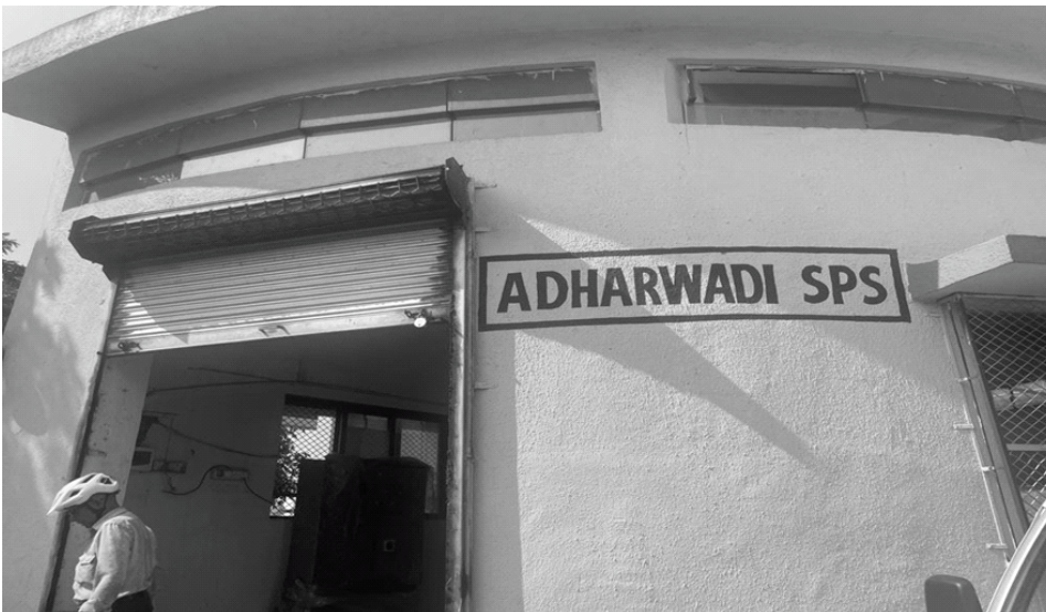
Site: Kalyan Sewage Treatment Plant, Aadharwadi Process Used: Sequential Batch Reactor (SBR)
